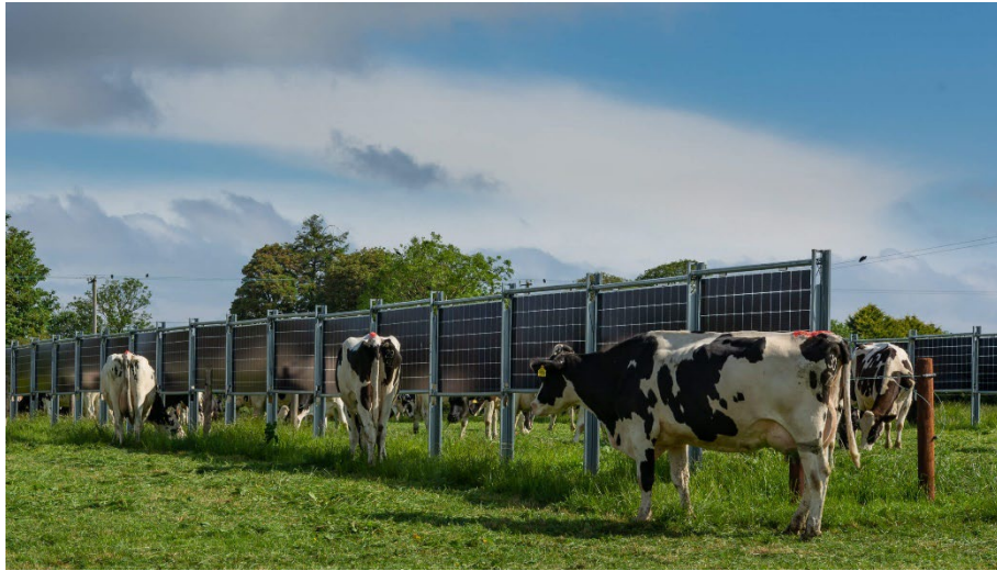
Vertical bifacial panels: Large animal grazing and hay production (Next2Sun, Germany)
